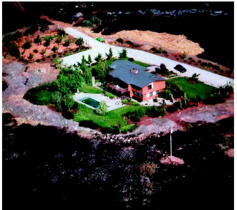
The pre-fire activities implemented by this homeowner included a green and well maintained landscape, reduction of wildland vegetation around the perimeter of the property, a fire resistant roof, and a good access road with a turnaround area. As seen in the photo, these pre-fire activities were effective.
